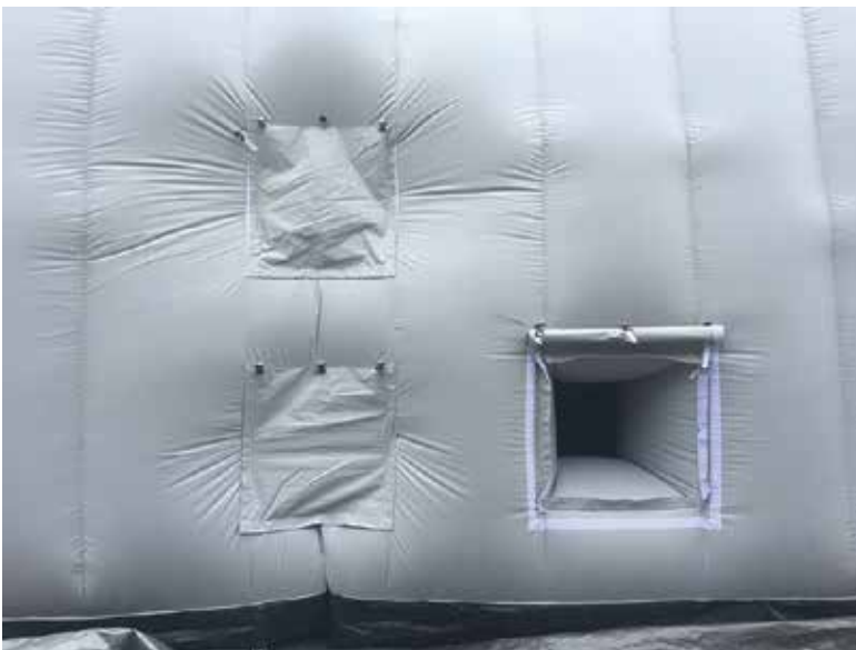
HVAC and exhaust fan ports
